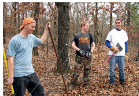
College Knights Jason Gangluff, Matt Winkeler and Aaron Isley repair a fence at the Clear Creek Monastery in Hulbert, Okla. Knights from four college councils — Cardinal John Henry Newman Council 7787 at the University of Arkansas in Fayetteville; Father Blaise Haritchabalet Council 5354 at St. Gregory's University in Shawnee; Oklahoma State University Council 11135 in Stillwater; and Tulsa University Council 11633 — gathered at the monastery to clean brush and perform other maintenance duties. Gangluff belongs to Council 7787, while Winkeler and Isley both belong to Council 11633.
